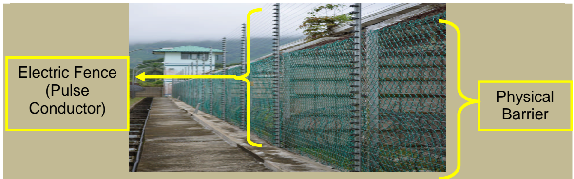
Figure 6: A physical barrier type based on a combination of chain-link (wire) at least 1.5 meter height. The pulse conductor is installed begins on the ground or physical barrier may be less than 1.5.
