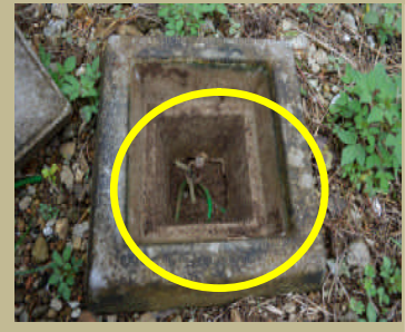
Earth Chamber (For earthing of lightning protection system)
